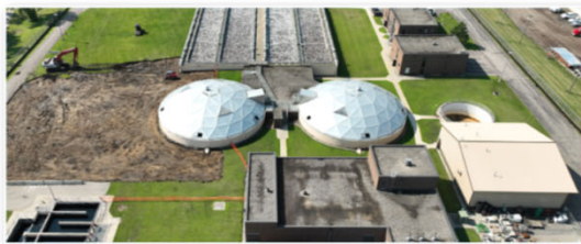
Owatonna Wastewater Treatment Facility
